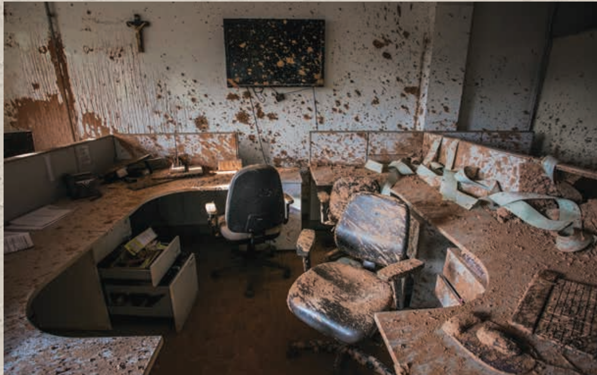
Management and command office at Vale's headquarters in Brumadinho, covered with mud
